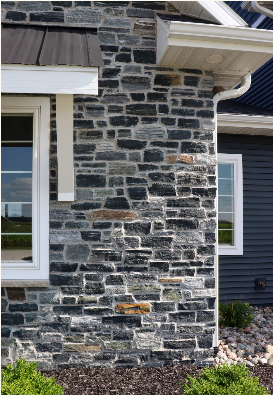
This wall owes its striking visual impact to a custom blend of 70 percent Black Frost Ashlar and 30 percent Barnwood Blue Ashlar—offering color notes from cooler charcoals and blues through warmer whites and tans.
